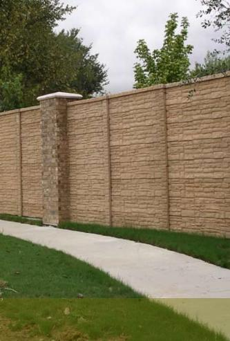
The fences simple design provides easy installation for contractors, landscapers and fence installers. The concrete posts are set into 12-inch diameter holes set five feet apart, posts are then anchored in a concrete footing. A bottom panel is then inserted down the post track and is supported by the concrete footing. Additional panels are stacked in one foot increments in an interlocking design.
